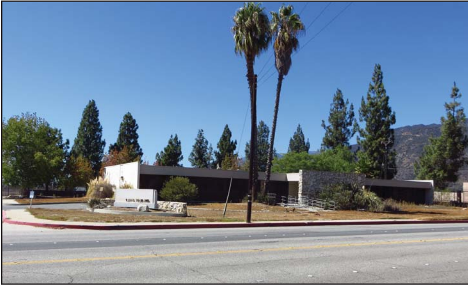
View of existing on-site office building adjacent to North Todd Avenue.
